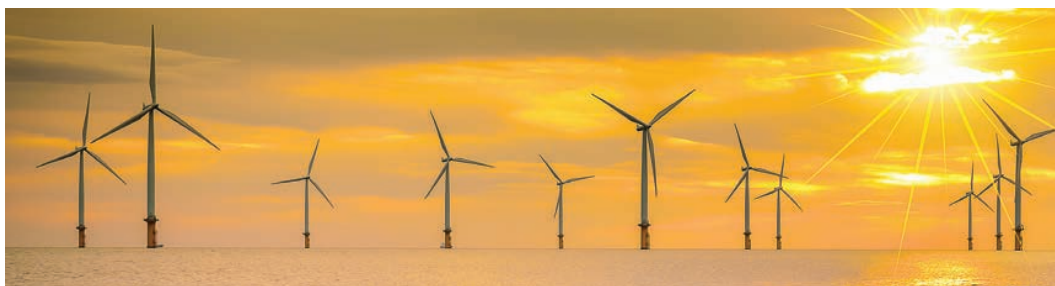
Left: Offshore wind farm in the UK
